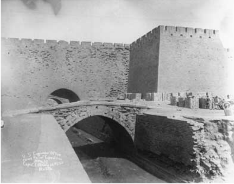
The sluice gate under the Tartar Wall.
