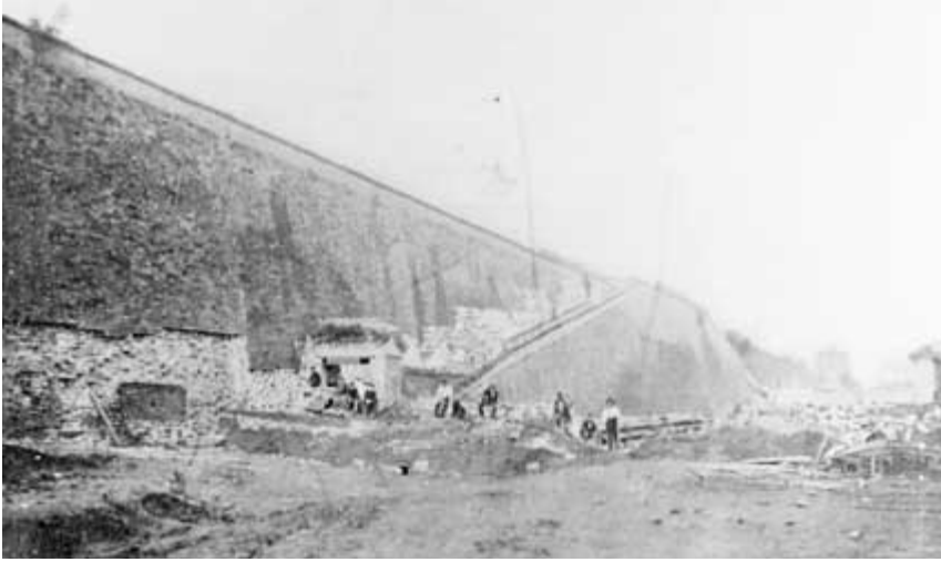
The ramp leading to the American position on the Tartar Wall.
